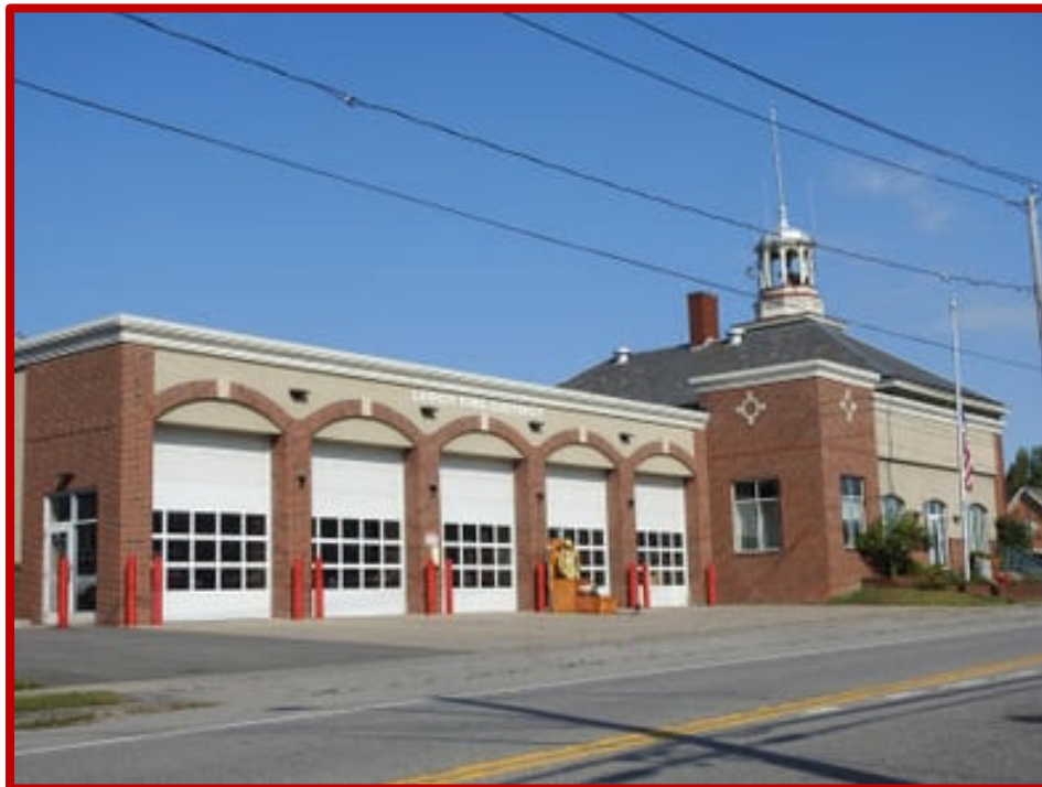
Figure X-5: LeRoy Fire District Fire Station Image credit: Firedepartment.net
