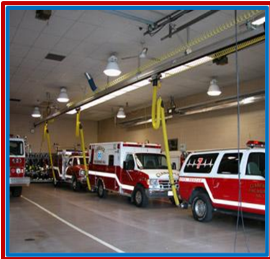
Figure X-7: Source capture vehicle exhaust systems can be utilized for both diesel and gasoline powered vehicles, and, can be attached to multiple vehicles parked in the same bay.
