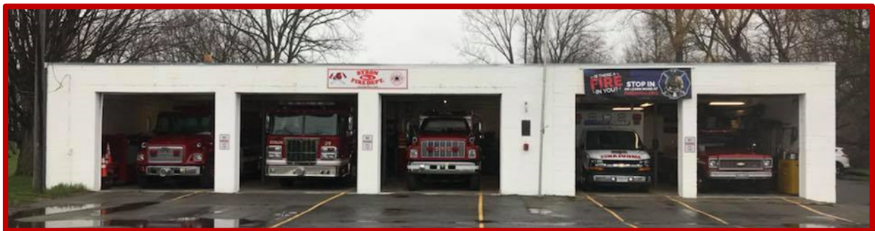
Figure X-2: Byron Fire Station
