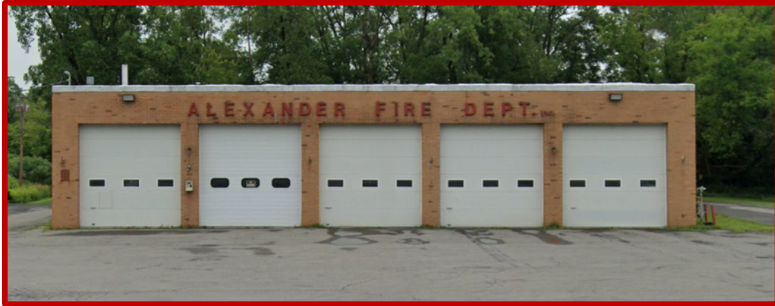
Figure X-1: Alexander Fire Station
